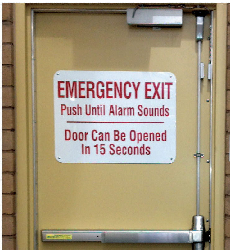
Figure 2. Principle of fail-safe defaults. This retail store keeps its back door closed and locked to prevent thefts. A “panic lock” allows the door to open during an emergency.
